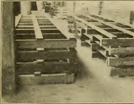
FIG. 1.—Crating on platform ready to load.
